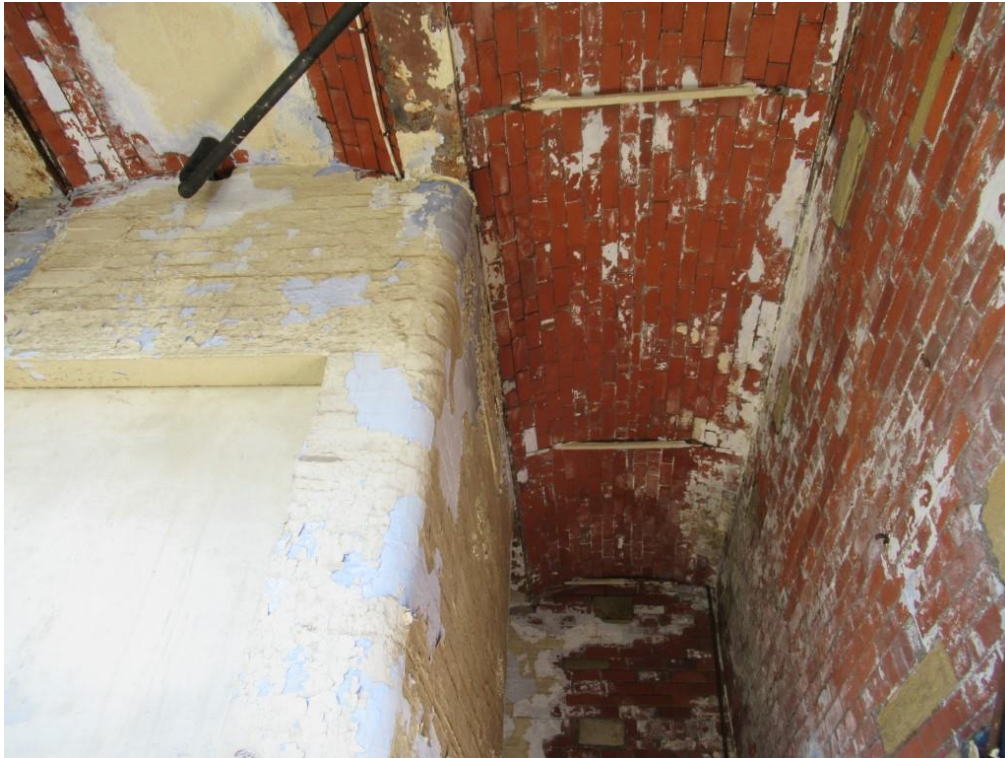
Photo 33 – Further view of the barrel vaulted ceiling, again in excellent condition.
