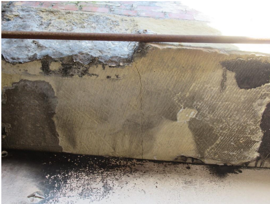
Photo 19 – Enlarged view of crack to the underside of the stone lintel – caused by fire damage, due to the intensity of the heat.
