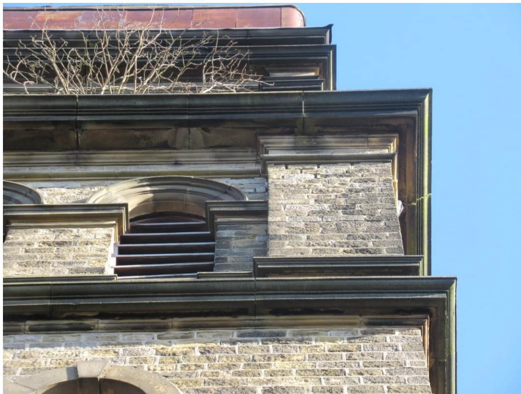
Photo 10 – Further open joints to corbelled stonework, above louvered bell tower opening.
