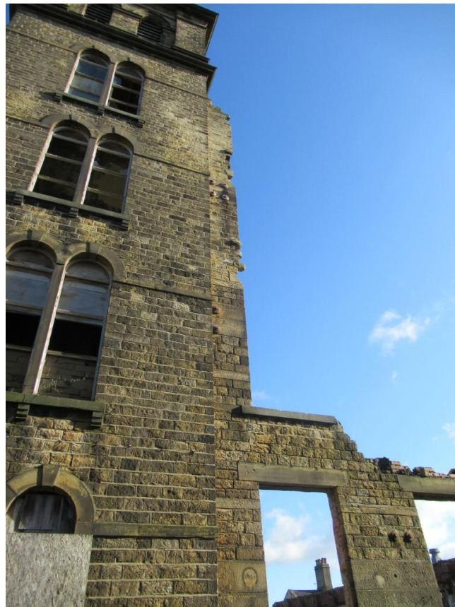
Photo 11 – Right hand side where the historical 4 storey high mill building, was previously attached. NB – Corner of the clock tower is perfectly plumb.
