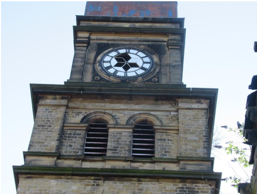
Photo 4 – Enlarged photo of top storey and 2 levels of corbelled stonework showing opening up of joints.
