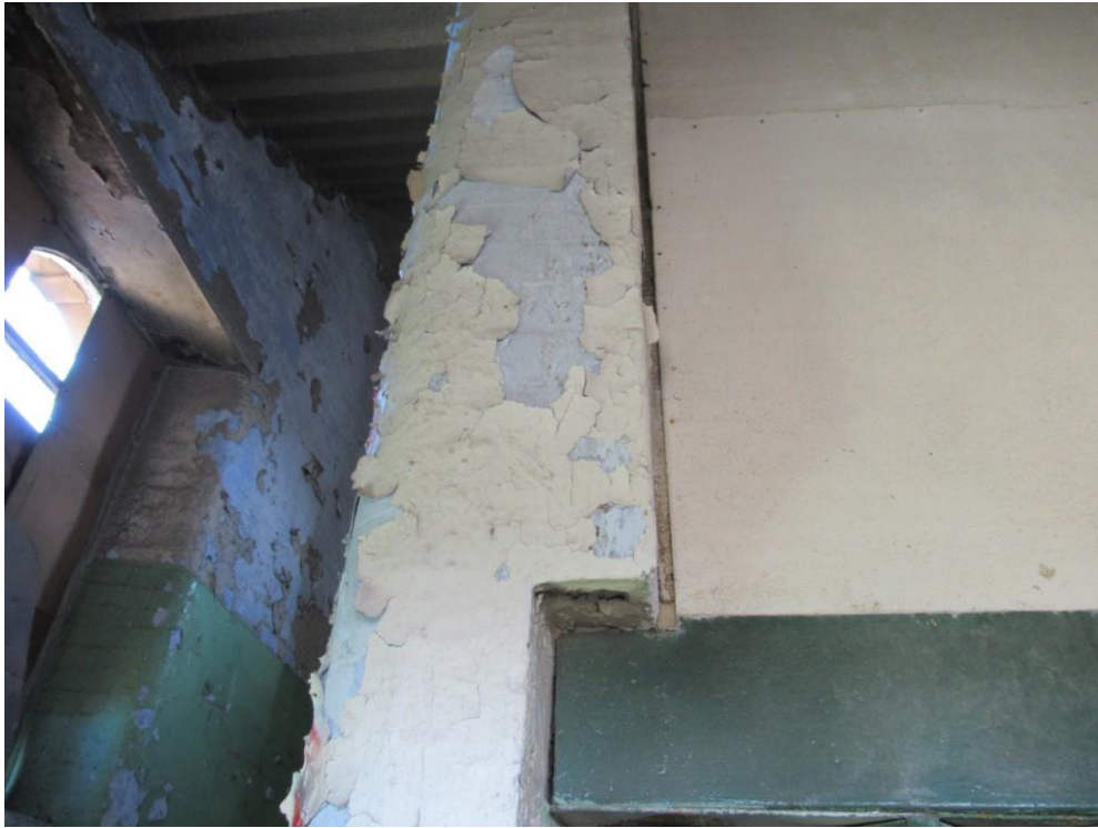
Photo 29 – Historical alteration to the width of the lift shaft. Typical at each level. Possibly required due to concertina action of retro fit lift doors.
