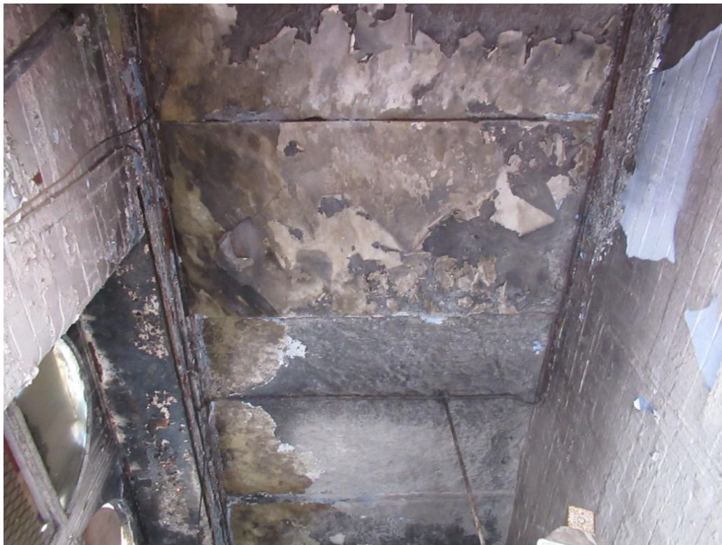
Photo 23 – Underside of fire damaged stone slabs to first floor landing.
