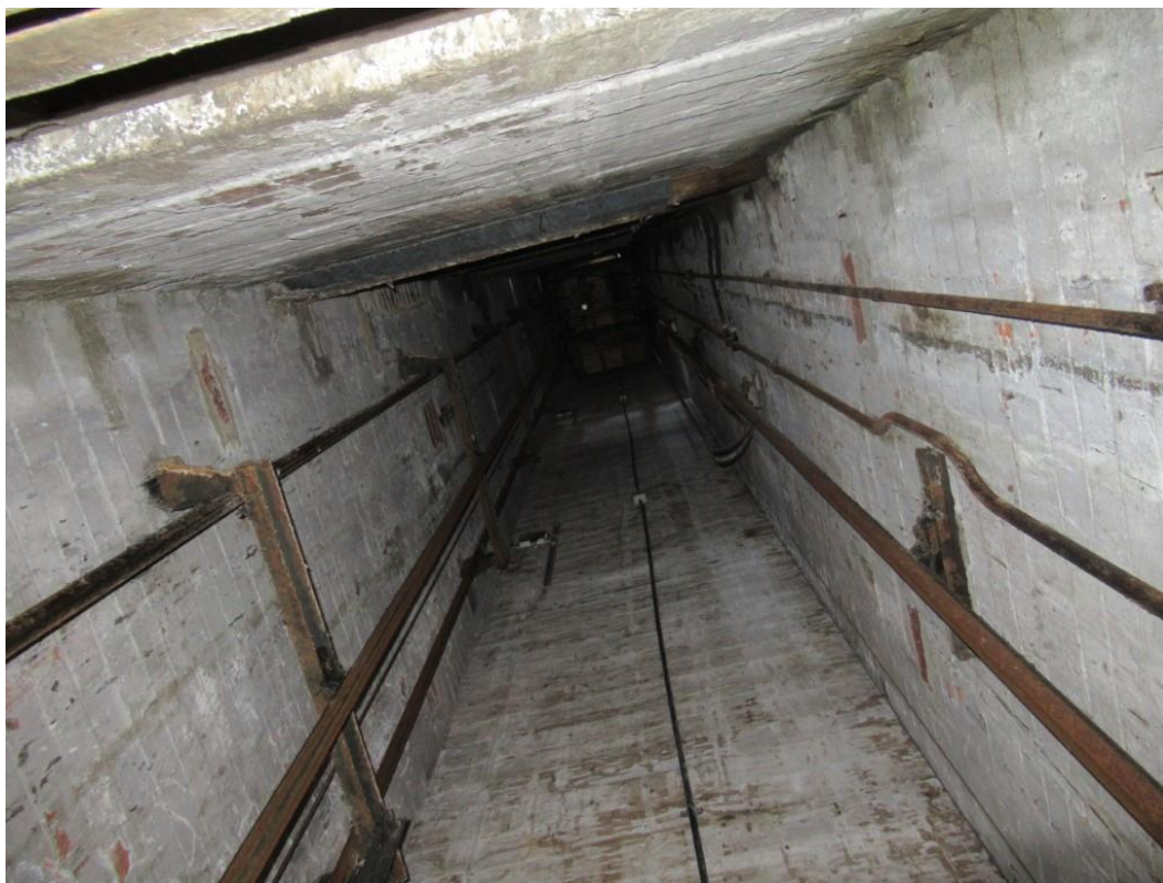
Photo 24 – General view of lift shaft. In excellent condition. All walls plumb.
