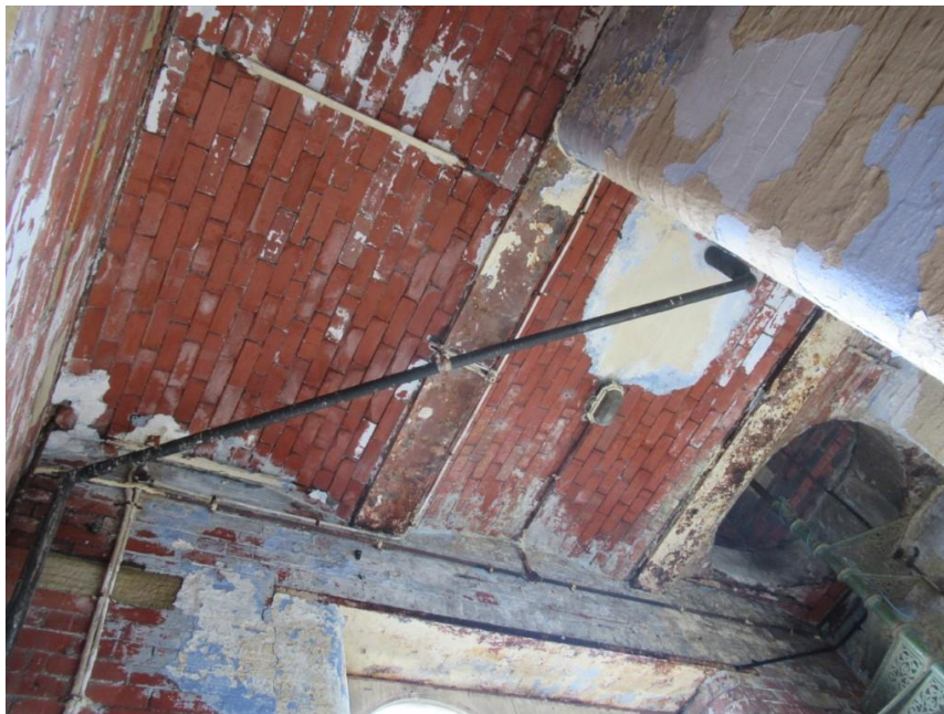
Photo 32 – Barrel vaulted ceiling to the third floor level, showing access hole for the spiral staircase to bell tower. Barrel vaulted brickwork is supported by cast iron beams with the rods present to prevent spread. Mild surface corrosion noted to the beams but otherwise in excellent condition.
