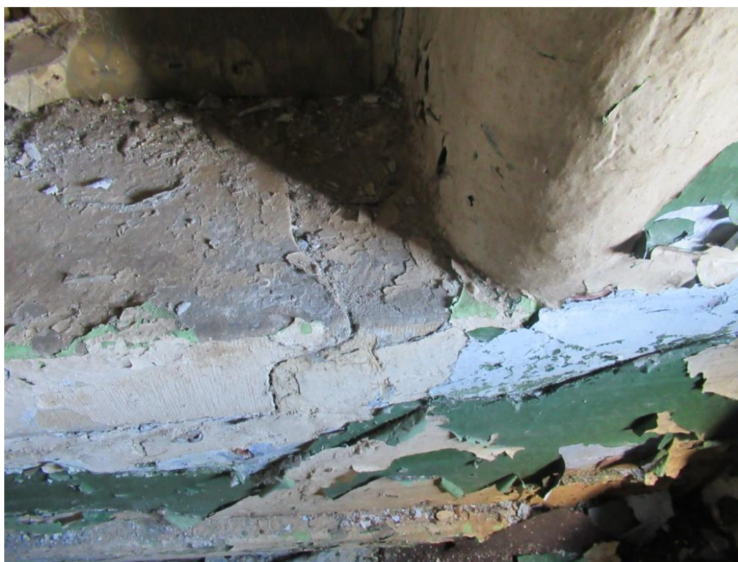
Photo 28 – Historical crack to window sill stone at first floor.
