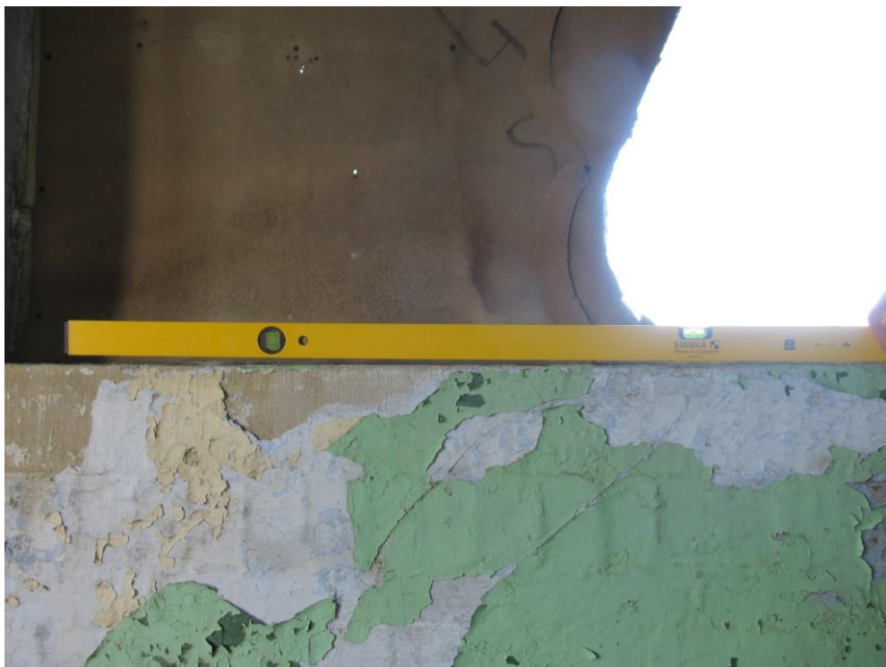
Photo 30 – Third floor sill stone. Possibly set incorrectly as no signs anywhere of any settlement or distortion of the clock tower building. NB, Levels were checked to the lift shaft brickwork and clock tower verticality in numerous locations with a 1.8m long spirit level and ALL found to be plumb with no lean.
