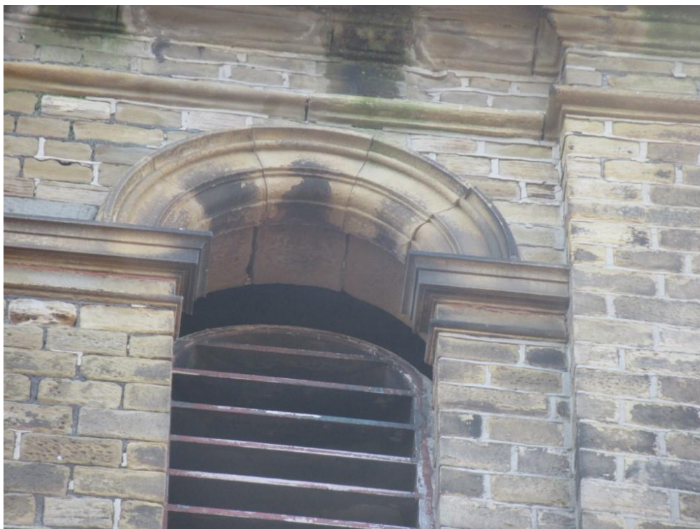
Photo 17 – Displaced corbelled stonework to arch, as right hand corner stone pillar has moved out. Timber louvre has become displaced.
