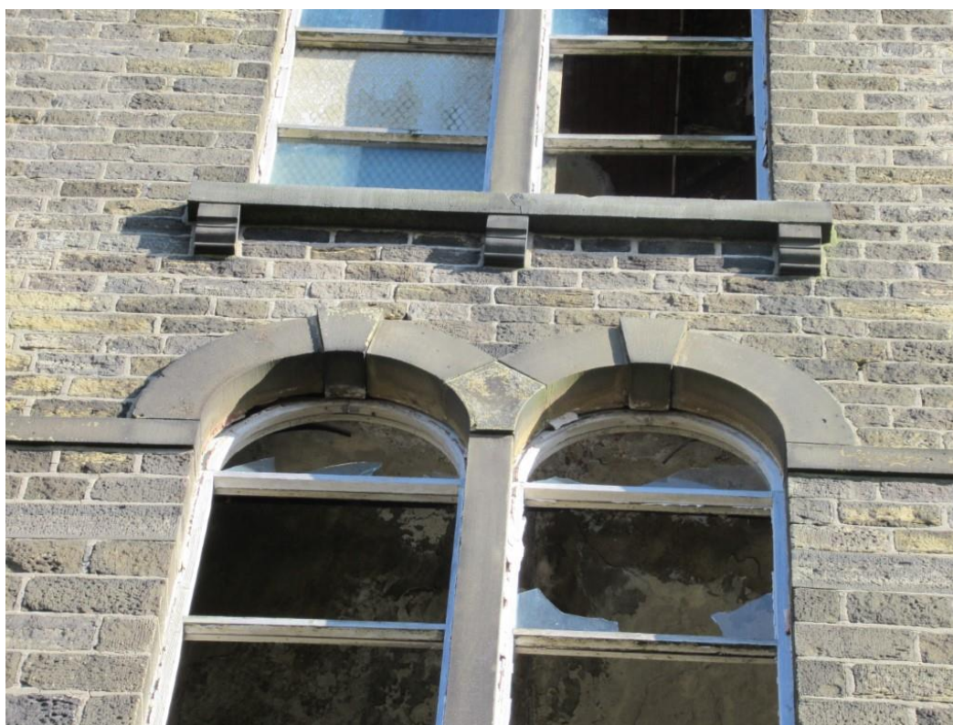
Photo 14 – General view of crack to third floor window sill.
