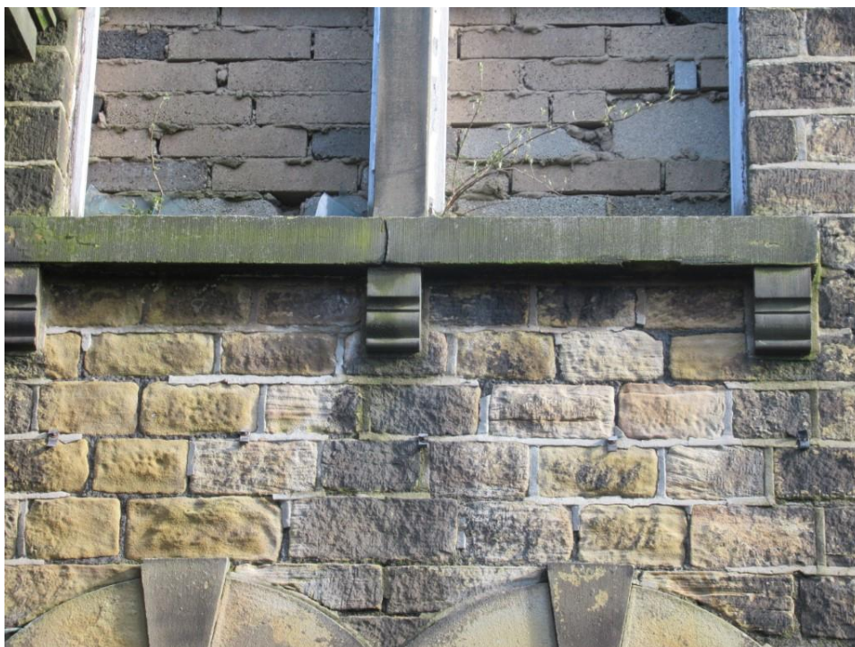
Photo 12 – First floor sill stone – Cracking at centre. NB , Localised loss of strap pointing.
