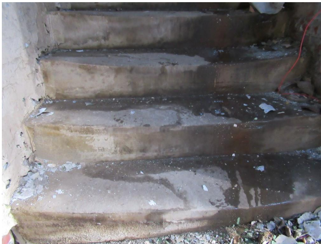
Photo 27 – Worn natural stone staircase flight, measured as 30mm of wear, but otherwise in excellent condition.
