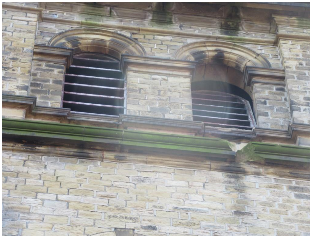
Photo – 16 – Enlarged view of fourth floor, showing impact damage to the stone corbelled course. NB Smoke damage as a result of the relatively recent fire.
