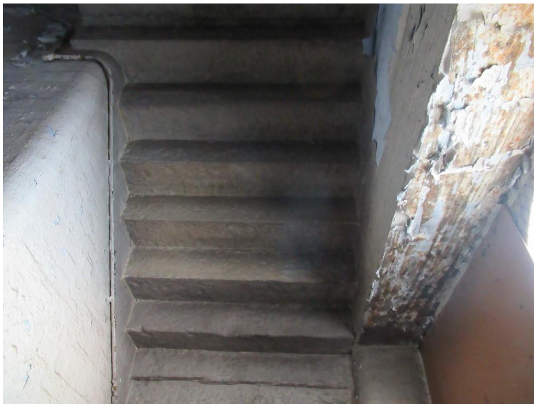
Photo 25 – Underside of staircase above ground floor quarter landing. Excellent condition.
