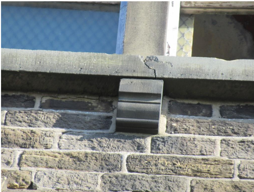
Photo 15 – Enlarged view of crack to third floor window sill.
