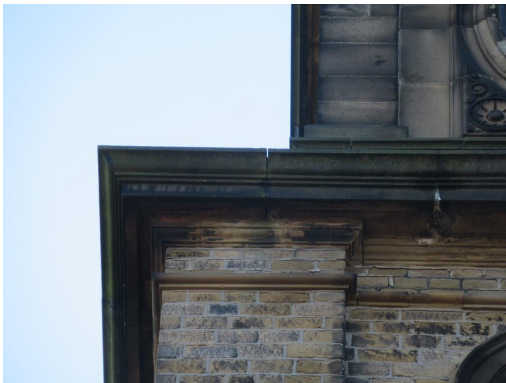
Photo 6 – Left hand side, showing further open corbelled stonework joints.
