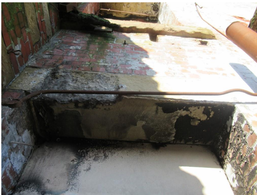
Photo 18 – Ground floor lintel – fire damaged.
