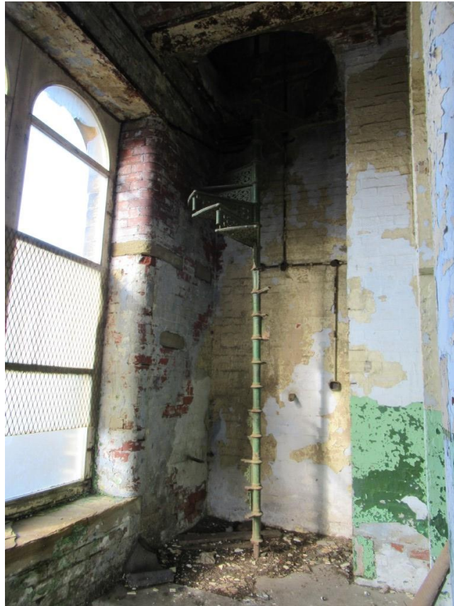
Photo 31 – Remains of the historical cast iron spiral staircase to the bell tower level.
