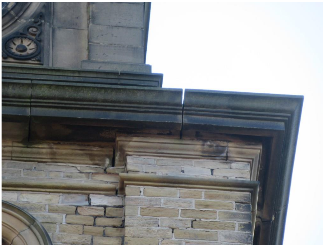
Photo 5 – Upper open joint to right hand side corbelled stonework – Also wide joints to bedded stonework, adjacent corner pillar.
