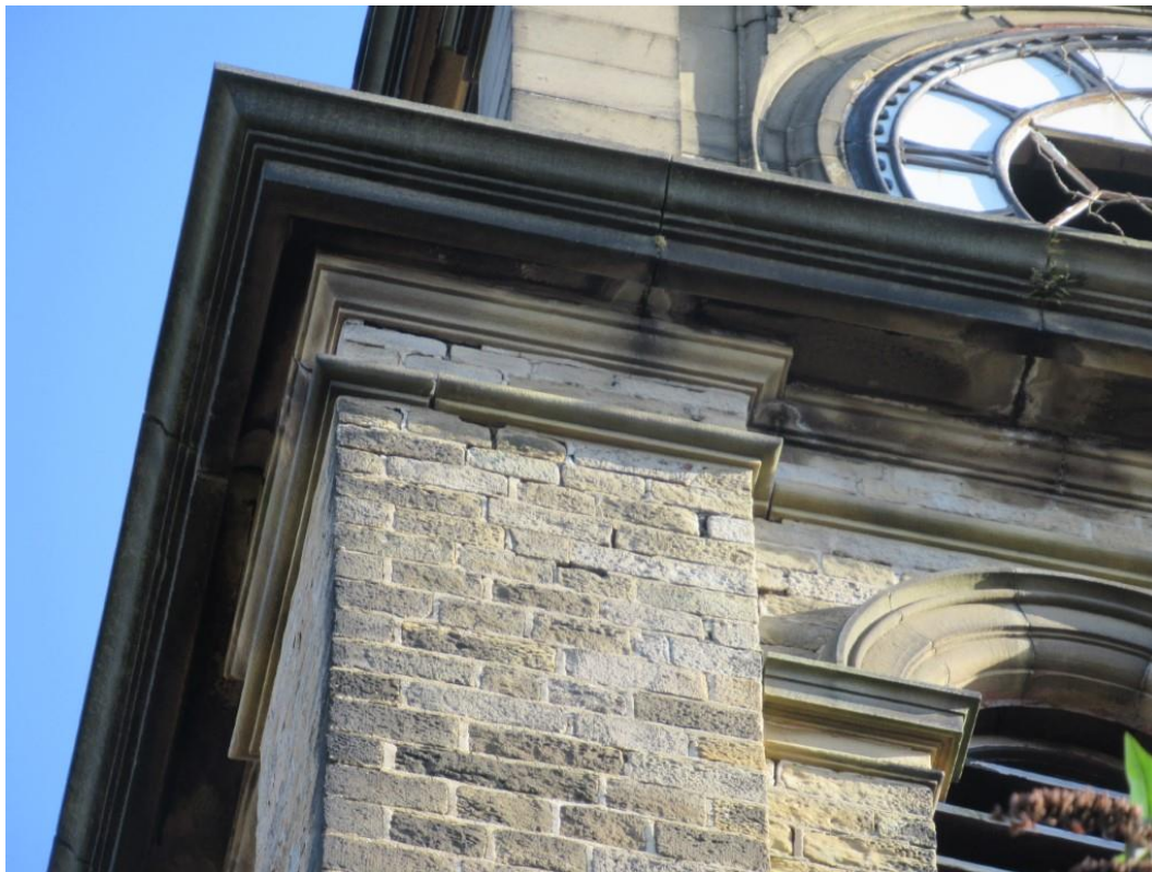
Photo 9 – Left hand side general open joints to walling stone at corner.
