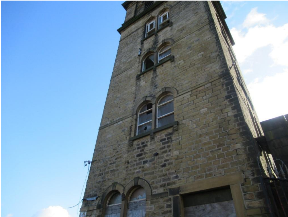
Photo 7 – Areas of strap patch re- pointing required.
